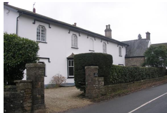
Fig.49 The Old Rectory: an elegant five bay late Regency house with interesting canted window heads. A remodelling (conversion from three estate workers dwelling according to the list description)
