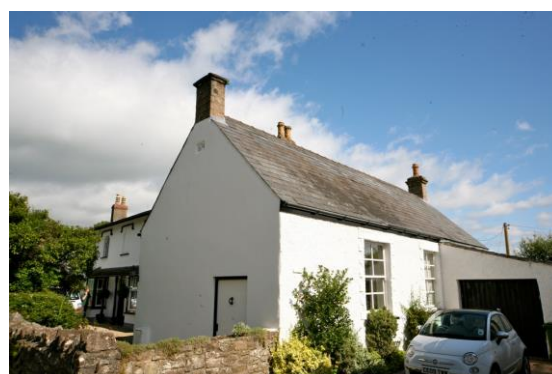
Fig.62 Natural slate roof to the Old Rectory
