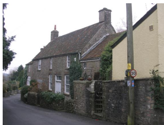
Fig.48 The simple vernacular form of the Old Meeting House, built in 1734-5, with its steep pitched roof and wide frontage, was probably adapted later to accommodate sash windows
