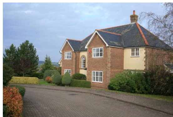
Fig.35 A typical house type at Redd Landes set in a landscaped cul-de-sac
