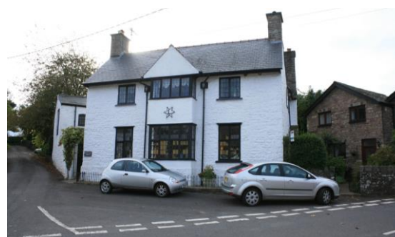
Fig.16 Newton Lodge probably by local architect Eric Francis
