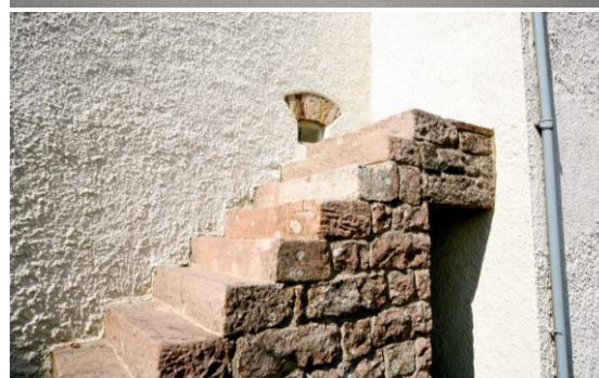
Fig.42 Mupper House (above) and its distinctive external stop steps (below)
