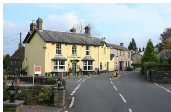
Fig.12 Tredegar Arms: positioned on a key corner site in the centre of the village
