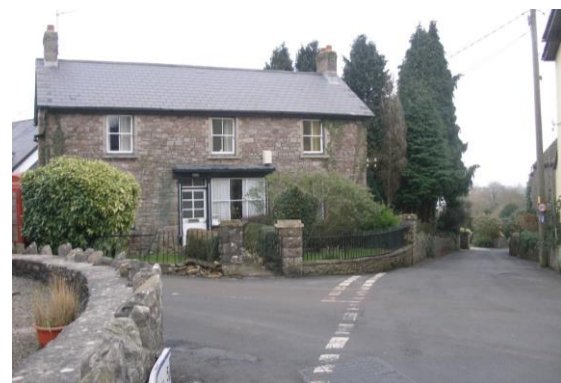
Fig.50 The former Post Office retains its 19 th century sash windows and shop window
