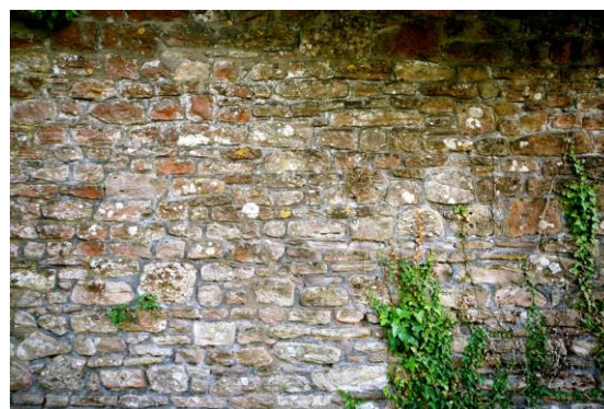
Fig.60 Typical colouration to the rubblestone walls
